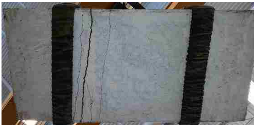
Figure 6.45. Crack pattern formation at the tension face of panel SUN3
