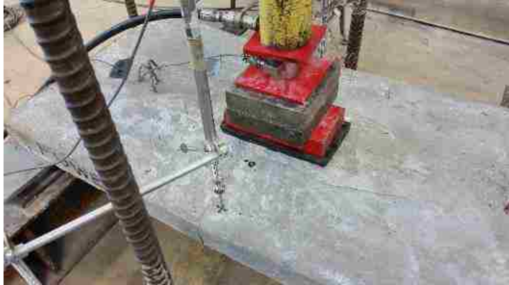
Figure 6.9. Panel FUC3 after failure
