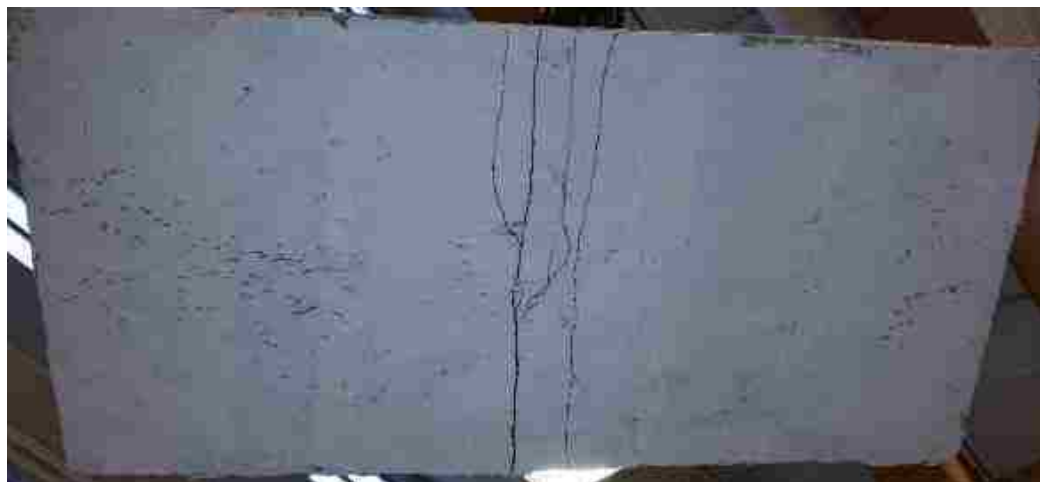
Figure 6.27. Crack pattern formation at the tension face of panel FUN2
