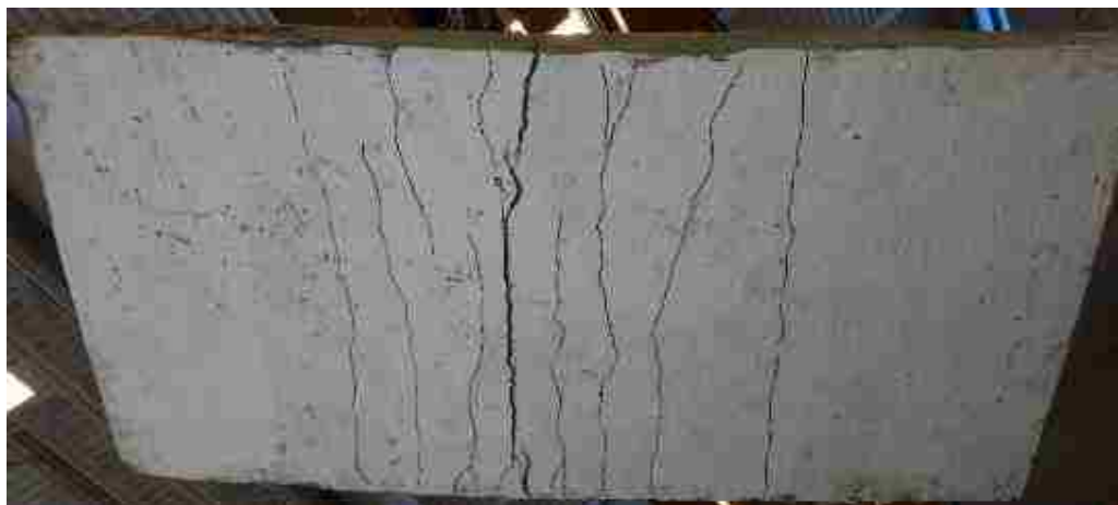
Figure 6.11. Crack pattern formation at the tension face of panel FUC3
