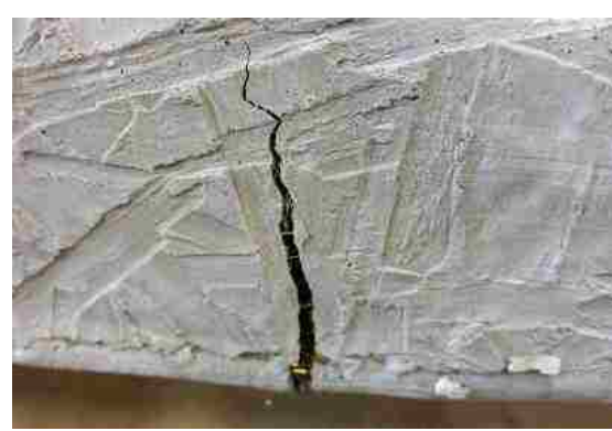
Figure 6.14. Tensile crack on panel FUW3
