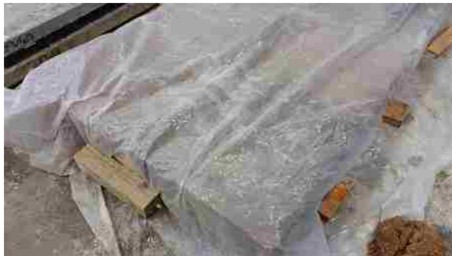
Figure 5.11. Plastic sheet on top of burlap
